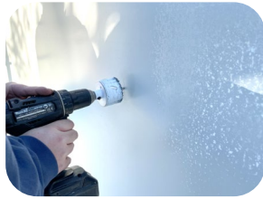
Bohren \varnothing 61 - 63
